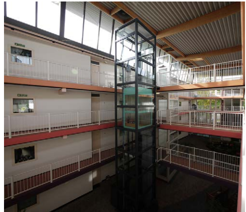
6.137 Vereniging AWDO Kreilerburcht, Rotterdam, The Netherlands A secondary lift had to be installed at considerable expense as the first one was not large enough for a stretcher or coffin.
