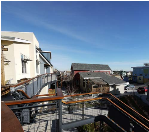
6.64 Silver Sage Cohousing, Boulder, Colorado, USA The external circulation causes problems in the cold Colorado winter climate where frost is common.
