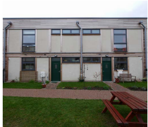
6.15: LILAC Cohousing, Leeds, West Yorkshire, UK The contemporary prefabricated design of LILAC Cohousing using a straw bale and lime render system called 'ModCell'.
